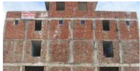
Figure 1(i) RC frame building with masonry infill (ii) short columns in the first floor
