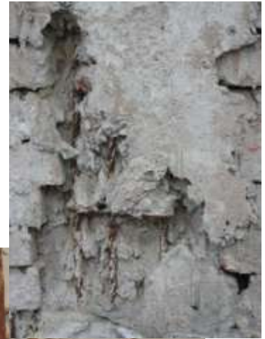
Figure 3. 90 degree hooks
