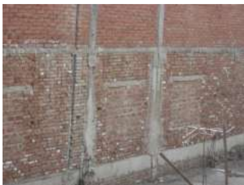
Figure 3. Pipe installation through beams and walls
