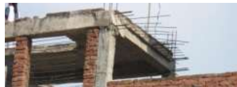
Figure 4 Poor beam column connections
