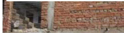
Figure 4 Poor beam column connections
