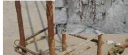
Figure 3. 90 degree hooks
